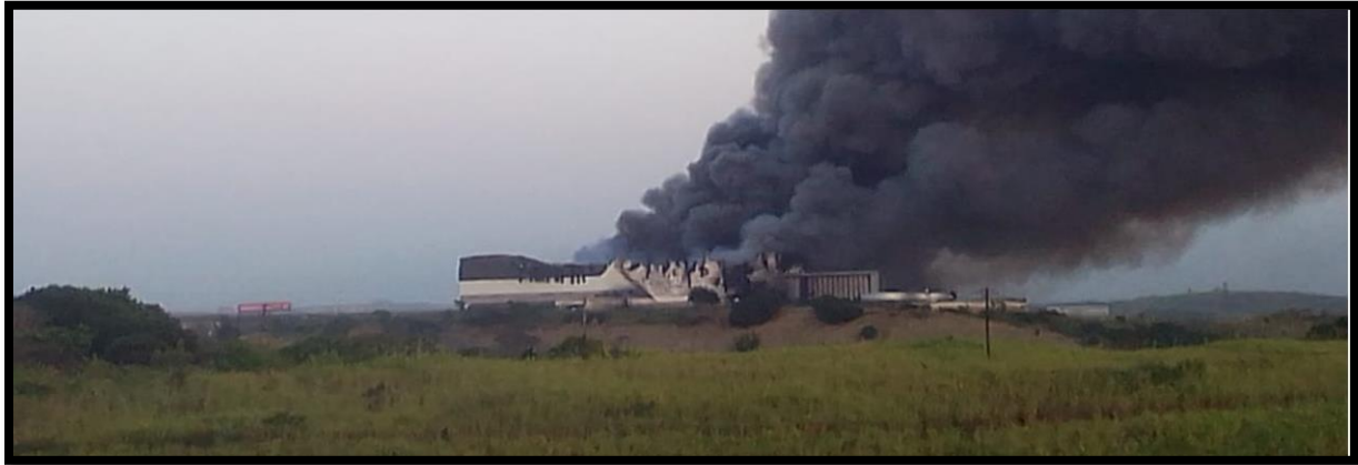
Figure 3.1: Fire after UPL Explosion (Mbele, 2021)
