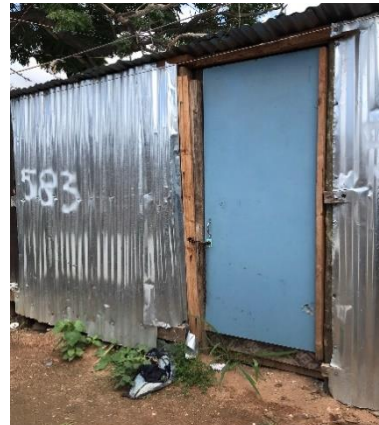
Figure 63 A typical informal dwelling unit. Source: Blanco, A 2021
