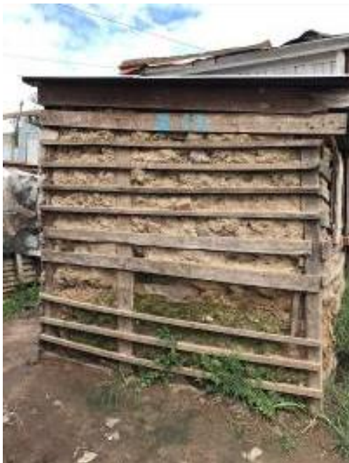
Figure 37 Earth-type construction method. Source: Blanco-Montero A 2022
