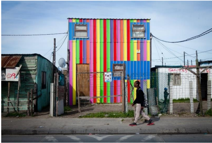
Figure 12 The external facade of a completed empower shack. Source:
