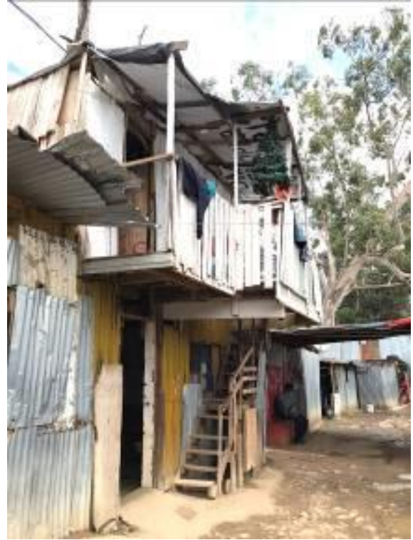
Figure 42 Staircase installed to enter upper floor of the dwelling. Source: Blanco-Montero, A 2022
