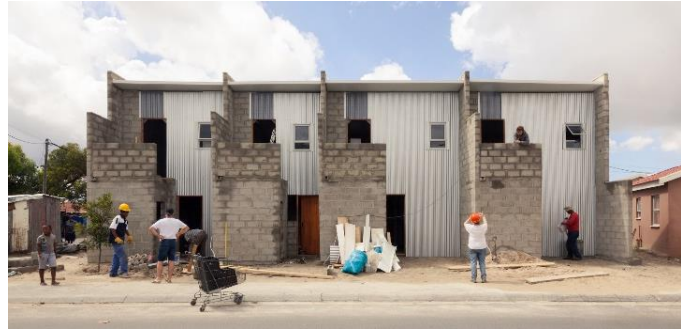
Figure 14 Empower shack 2.0 construction out of more durable material. Source: https://uttdesign.com/works/empower-shack--6
