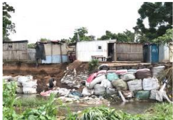
Figure 44 Sandbags on the river bank used as a retaining wall. Source: Blanco-Montero, A 2022
