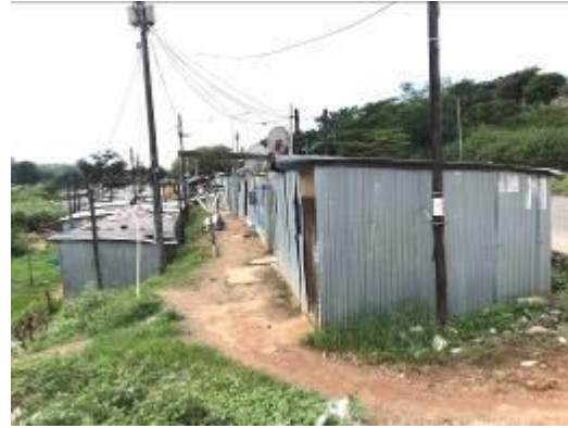
Figure 40 Legal electrification in Mampondweni.
