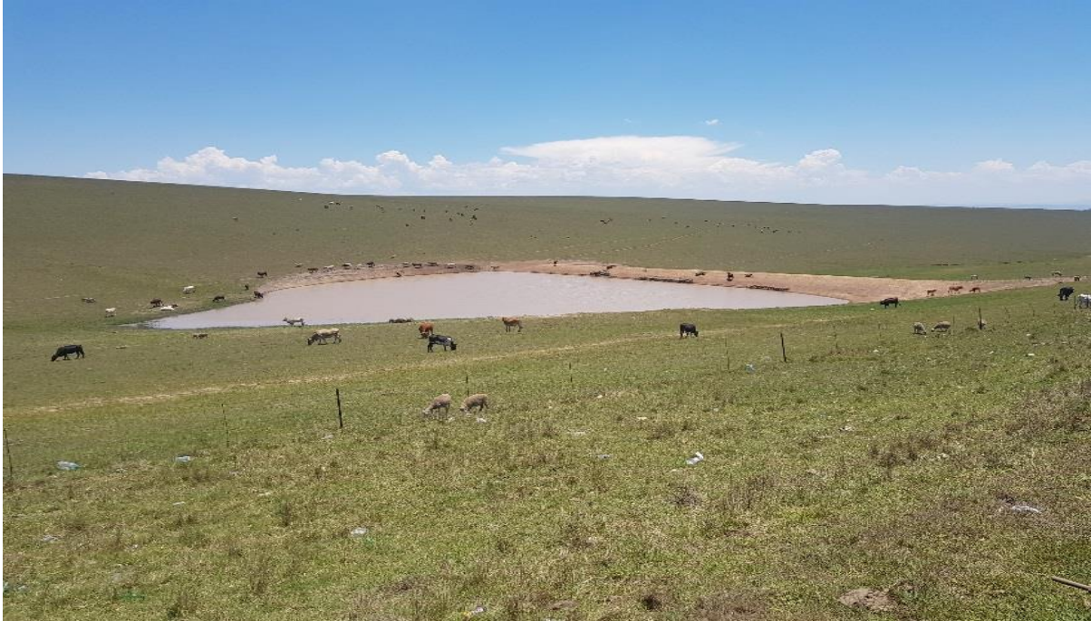
Figure 15: Typical well-rehabilitated dam in Sidwadweni in Tsolo
