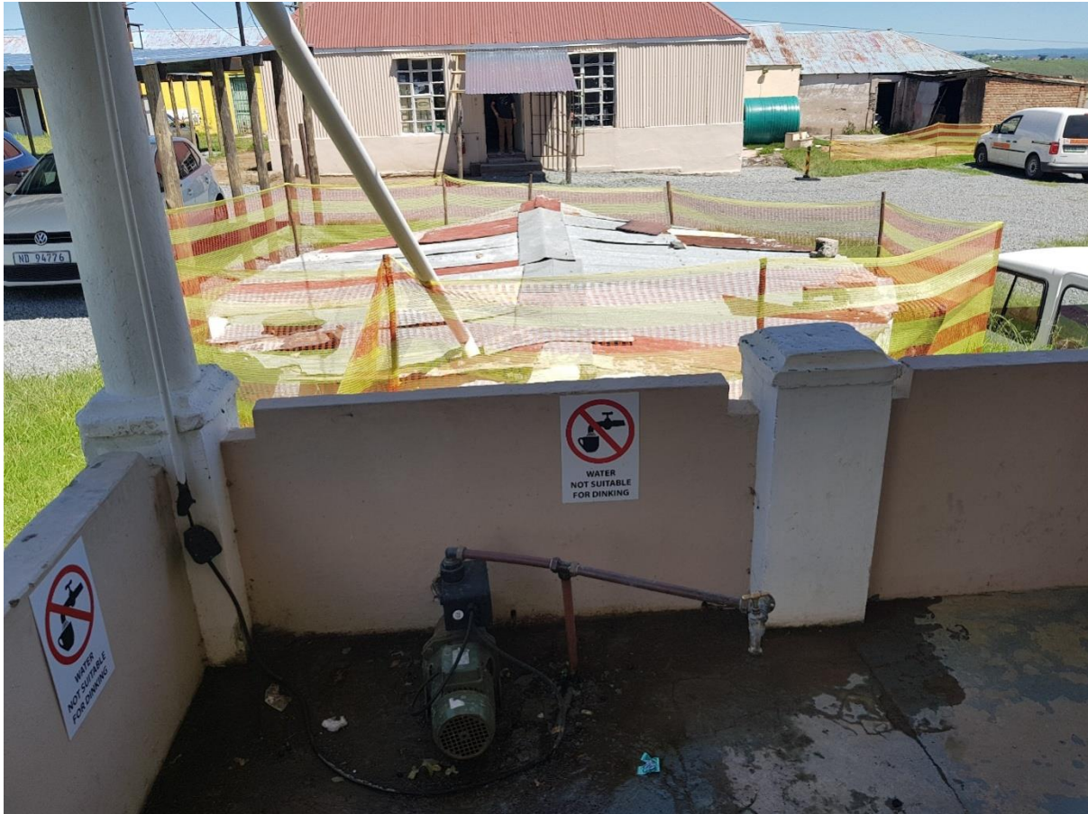
Figure 24: Underground water in a local guest house in Ndabakazi village
