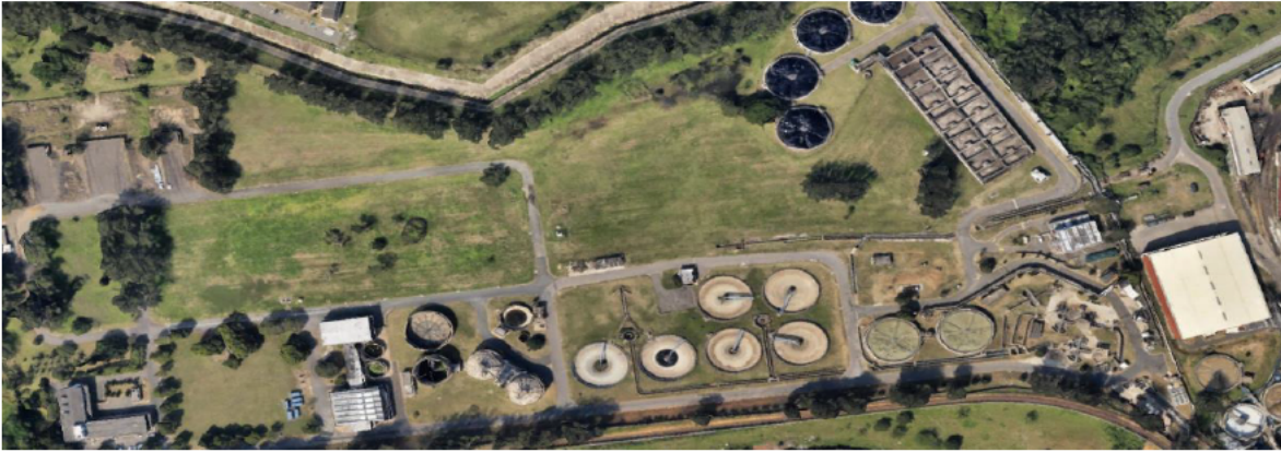
Figure 3-2: Ariel view of the municipal wastewater treatment site supplying with activated sludge
