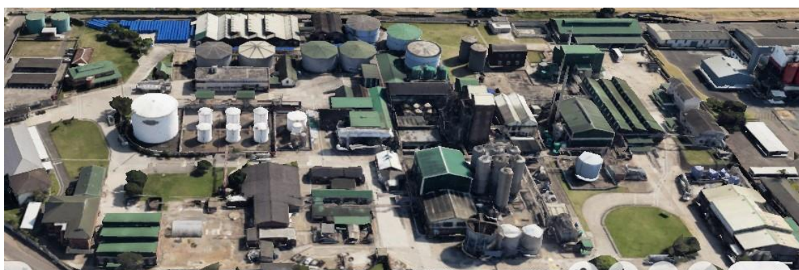
Figure 3-1: Ariel view of the sugar refinery site supplying with the effluent
