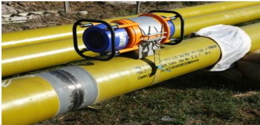
Figure 2.3: Inspecting pipelines using the RT Technique (Global Welding, 2025)
