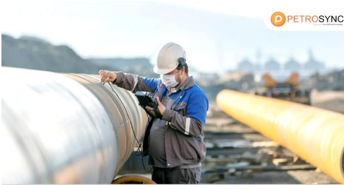
Figure 2.2: Inspecting pipelines using the UT Technique (petrosync, 2025)
