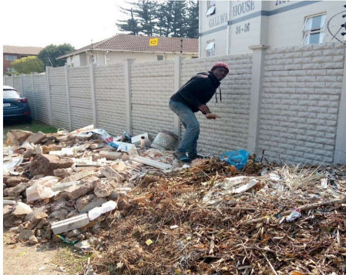
Figure 3.5: Ceramic wastes dumped on a site in Pietermaritzburg (Photo by Peace Adedeji, taken at Pietermaritzburg, 2023)
