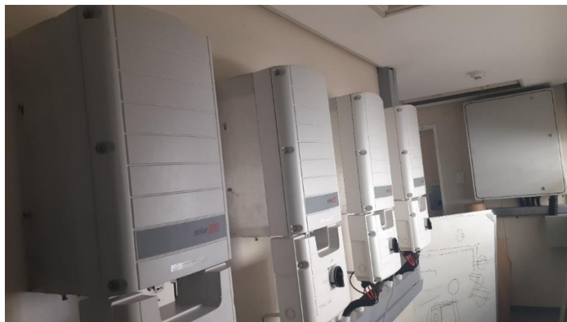
Figure 4.18 The three-phase inverter
