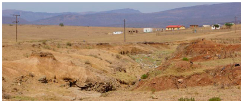
Figure 1. Land eroded by heavy rains in Cofimvaba. The degraded land can no longer be cultivated. Source: Meyiwa et al
