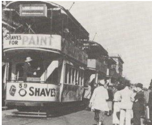
Figure 3.5: Electric double-decker jammed due to power failure (Morrison 1987:33)
