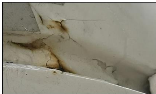
Figure 2:2. Formation of filiform corrosion.
