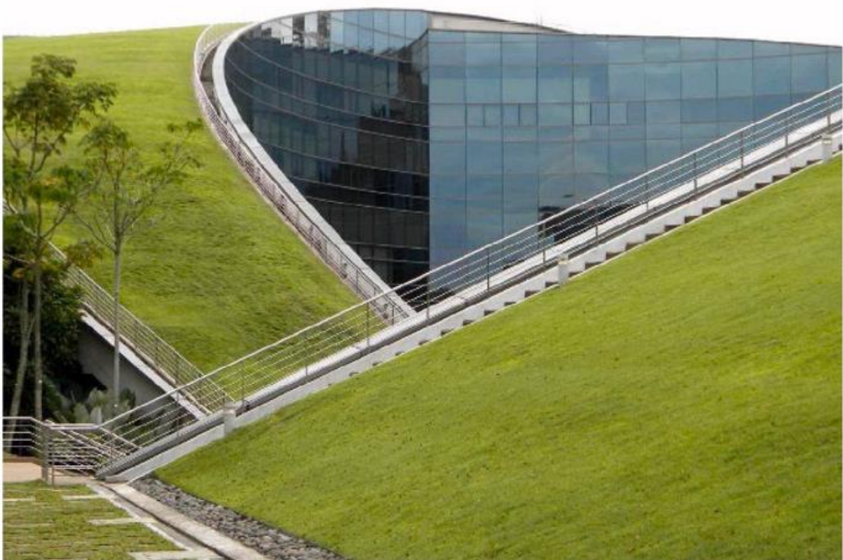
Figure 2.5: Nanyang Technological University's green roof in Singapore (Lai et al. 2023)
