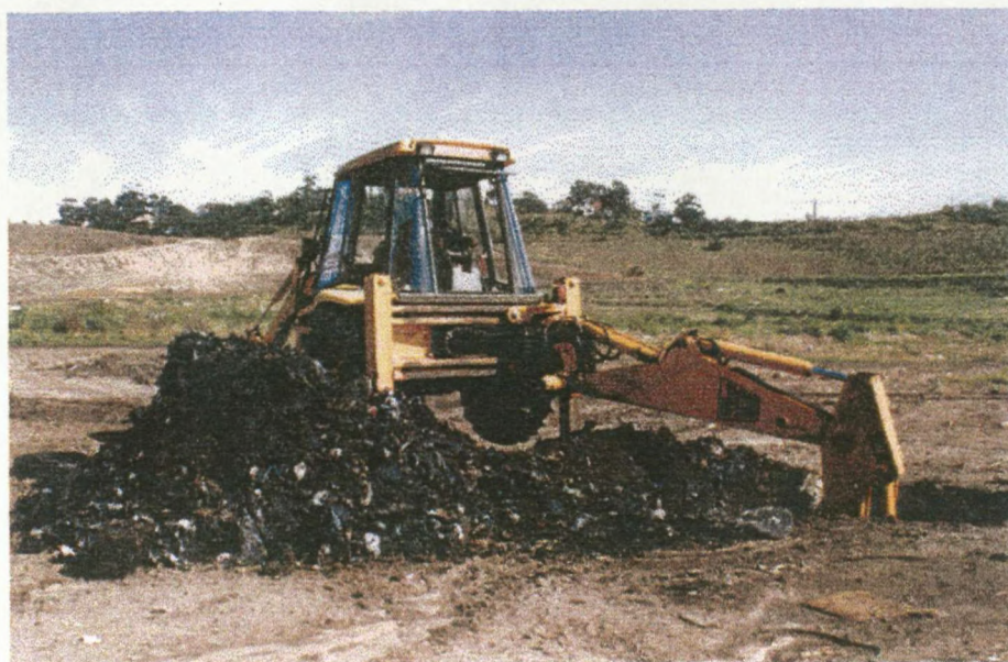
Figure 4.2 Excavation for sampling
