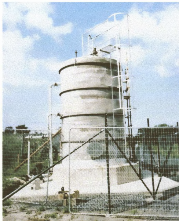
FIGURE 2.8 Pilot-scale bioreactor containing Cr(VI) reducing organisms (Turick, 1997).
