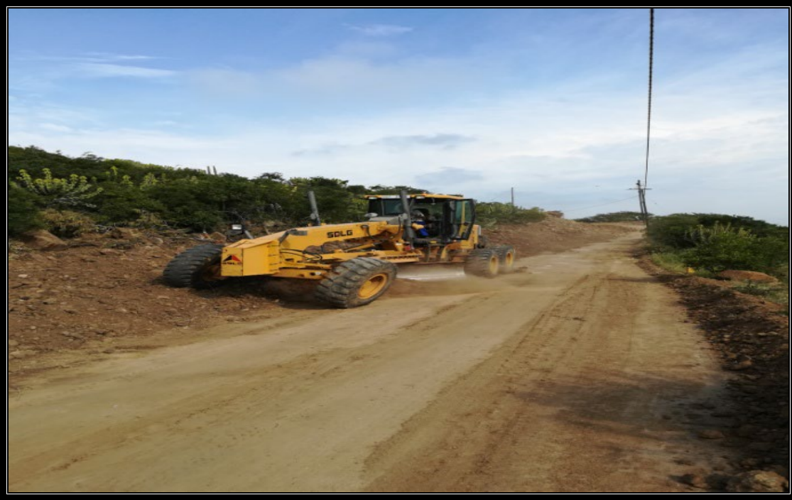
Figure 4. 3. Rip, spreading an cutting of levels with grader on road D1264 in 2013
