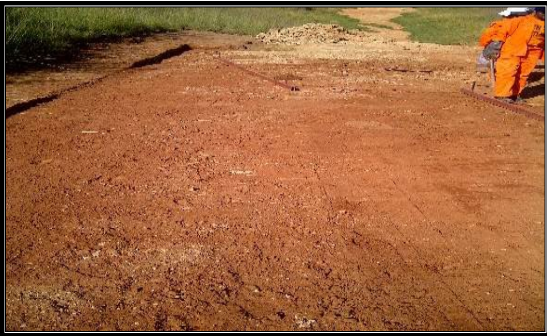
Figure 4. 2. Camber formation before compaction on road D1264 in 2013
