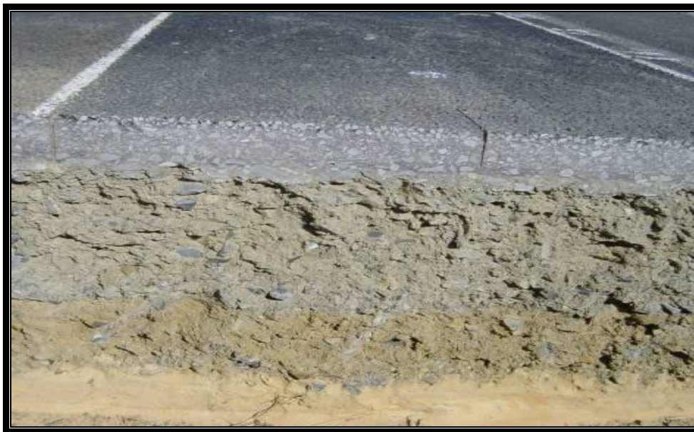
1. Figure 2. 2. Road cross-section showing road layers (SANRAL,2014)
