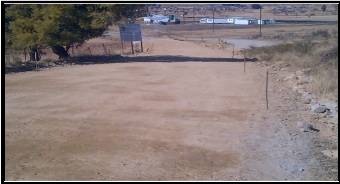
Figure 2. 7. A TMM completed section on road D1264 formation layer
