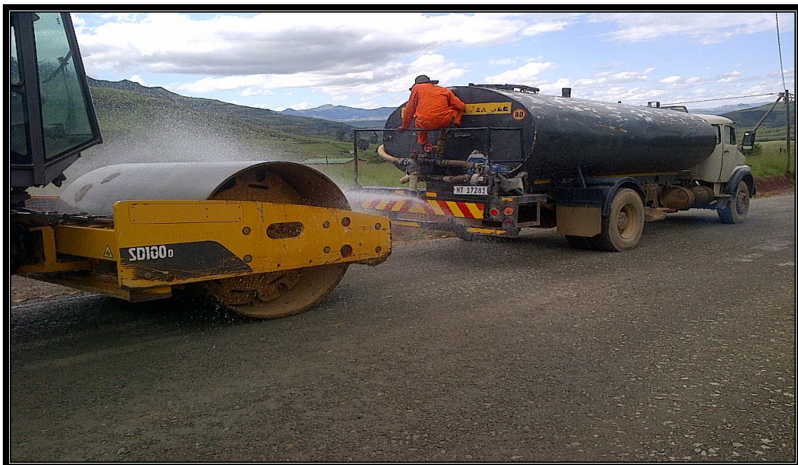
Figure 2. 4. Water cart and smooth roller during Road D1264 road construction in 2014
