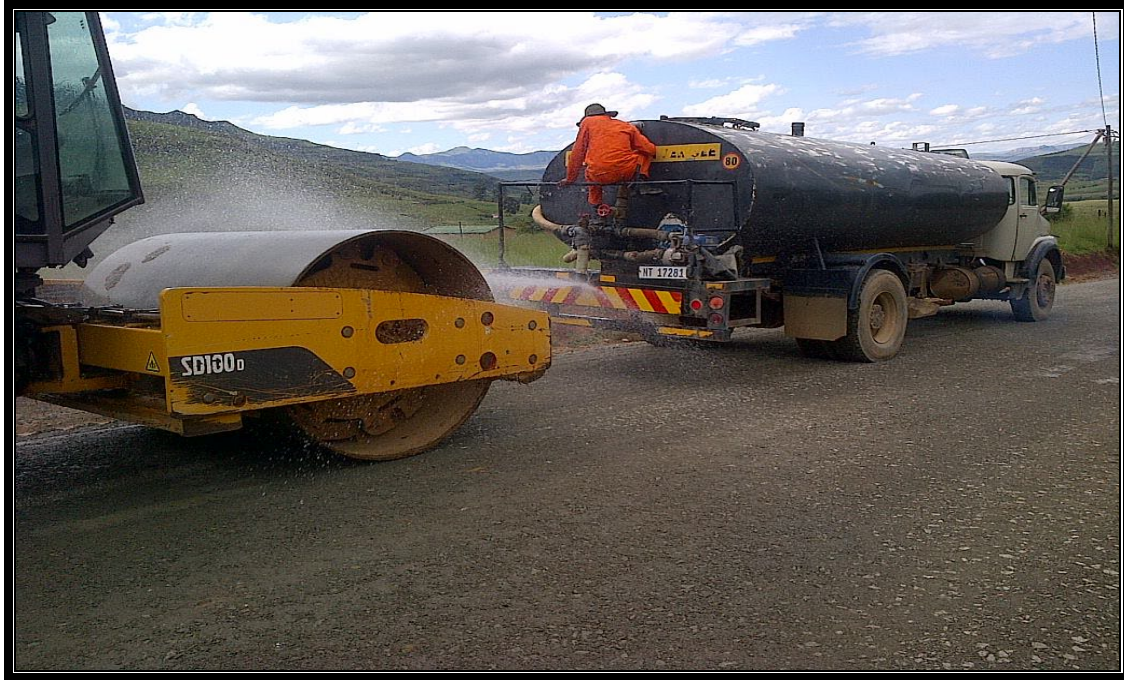
Figure 4. 5. Compaction using smooth roller and water cart on road D1264 in 2013
