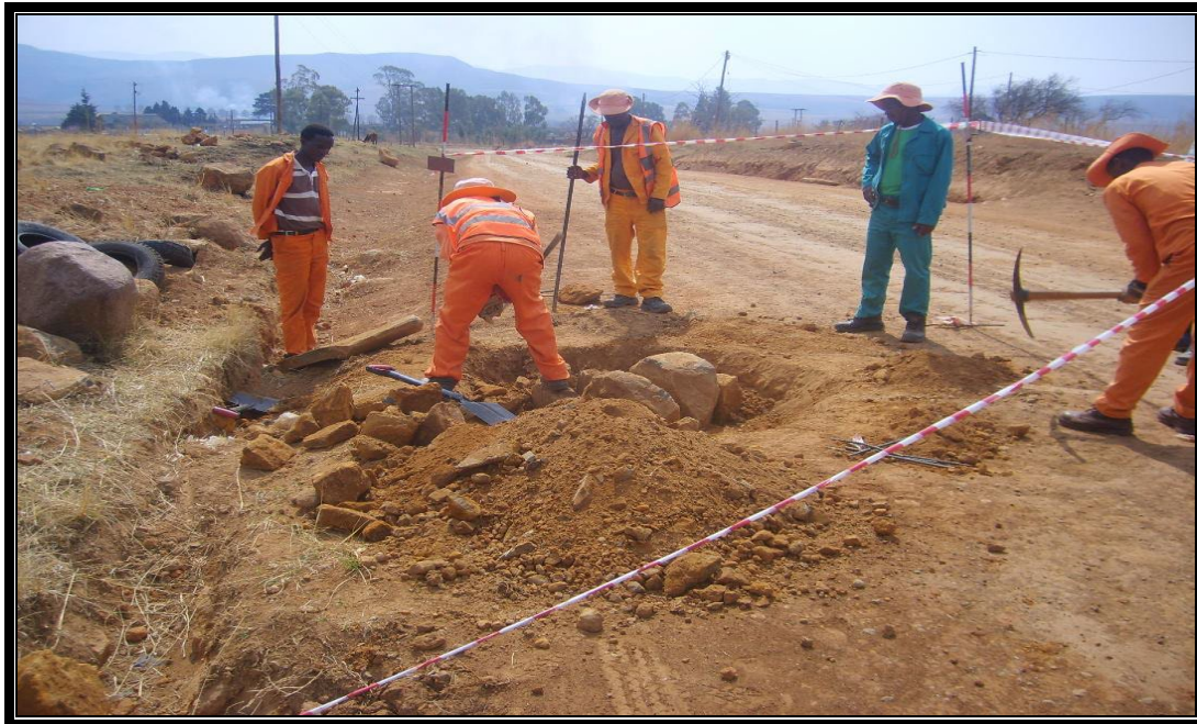
Figure 1. 1. Excavation using LIC during the formation construction on Road D1264 in 2013
