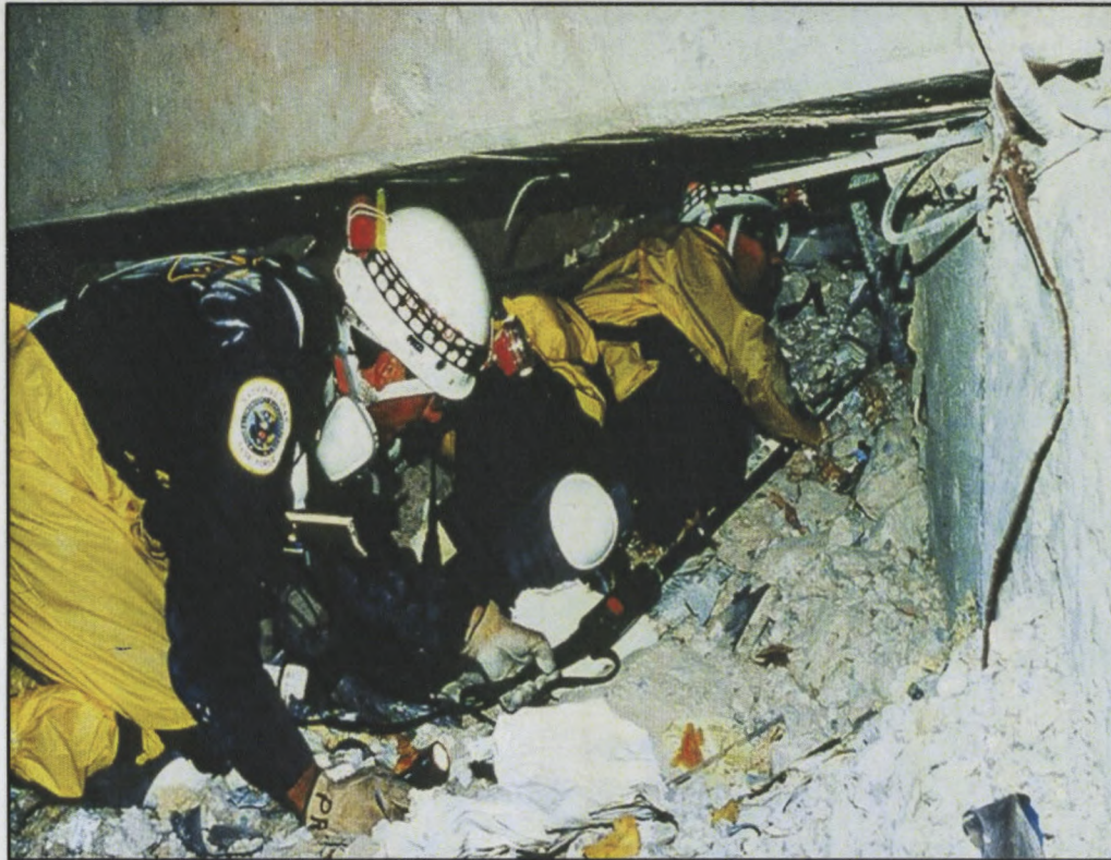
Plate 2-3 USAR work in a confined space inside a collapsed structure (OCHA-FCSS, Real time)
