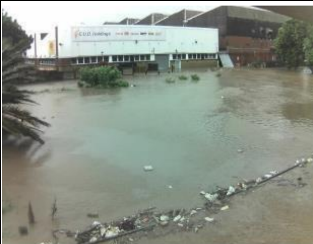
Figure 28: Toyota Canal Hiace Gate 1
