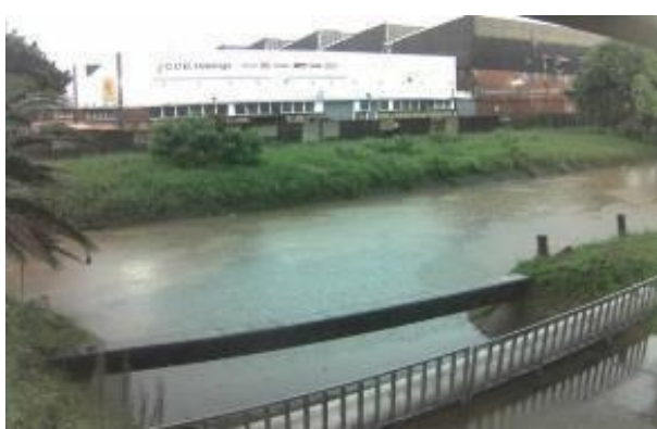
Figure 26: Toyota Canal Hiace Gate 1
