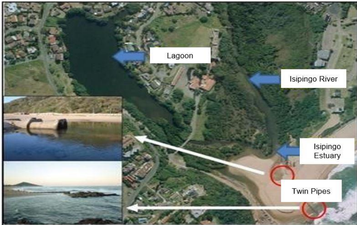
Figure 19: Two x 1m diameter concrete pipes for tidal exchange.
