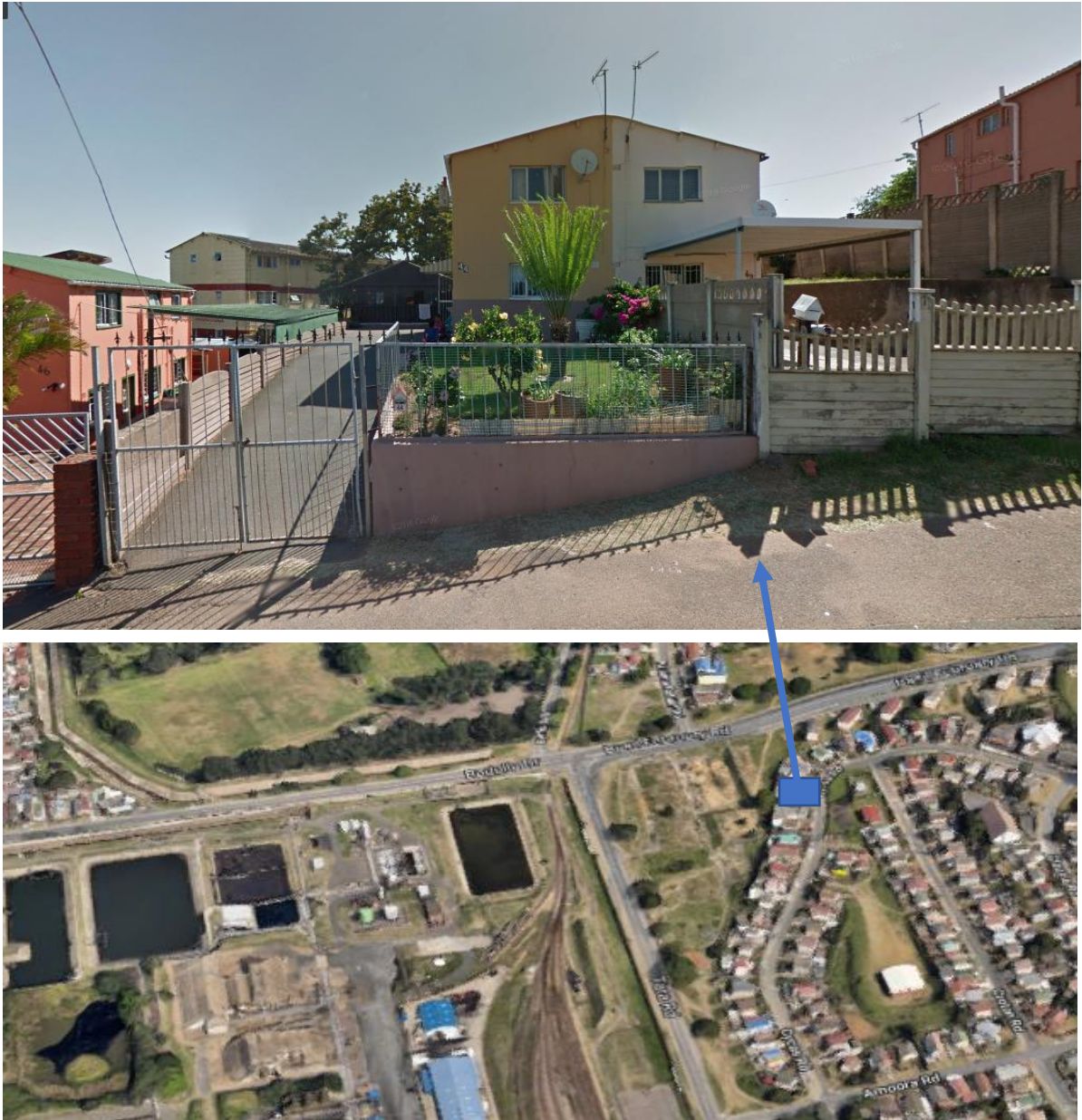
Figure 20: An example of HBE typology and layout in Austerville (Image created by author using aerial view from Google Maps, 2019)
