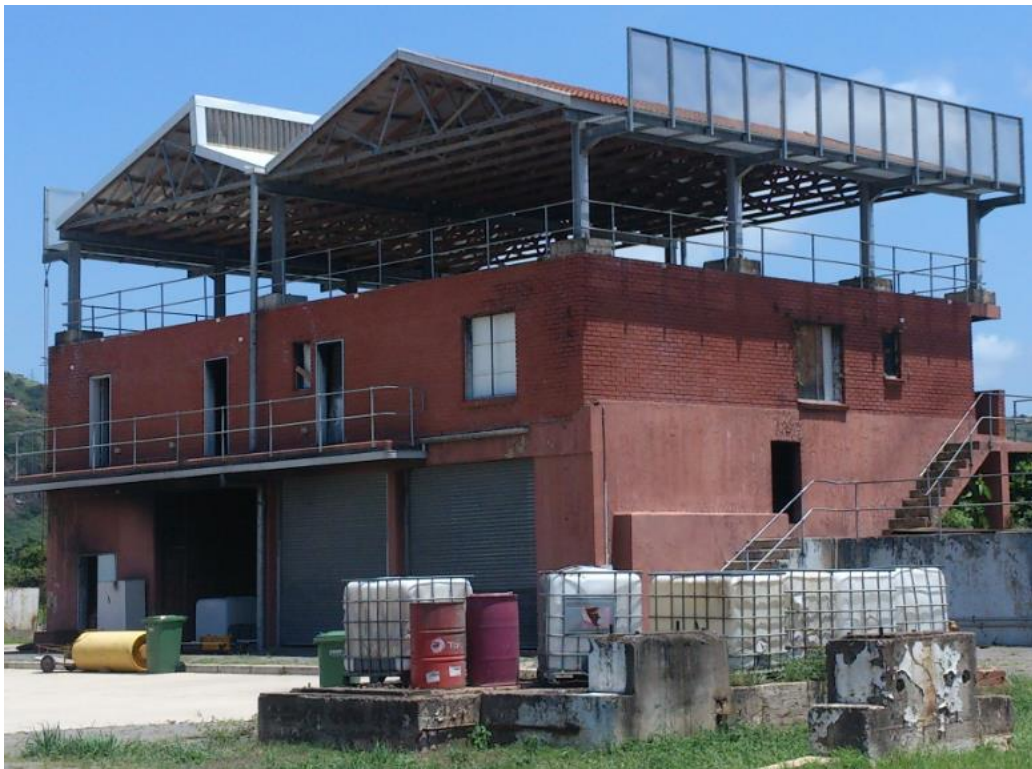
Figure 11:eThekwini live fire training structure
