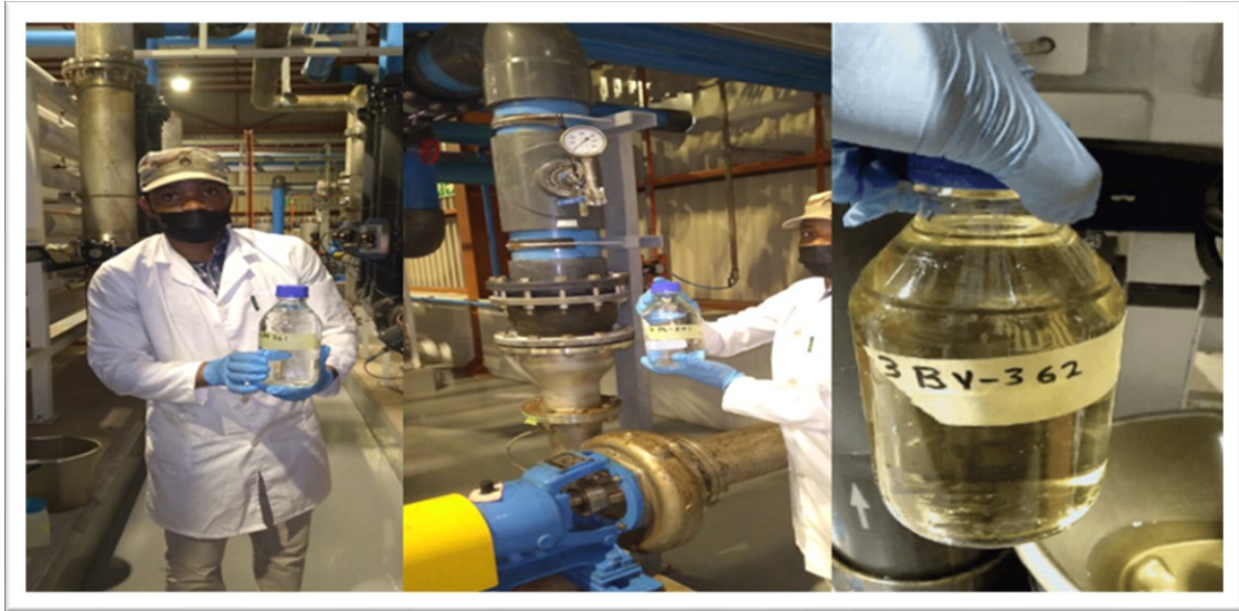
Figure 3.4 Depiction of water samples collection at the REMIX Water Treatment Plant.
