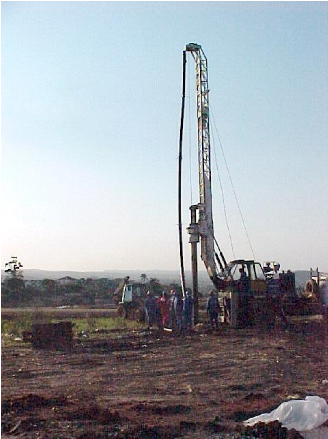
Figure 12: The Process of Insertion of Vertical Extraction Pipes
