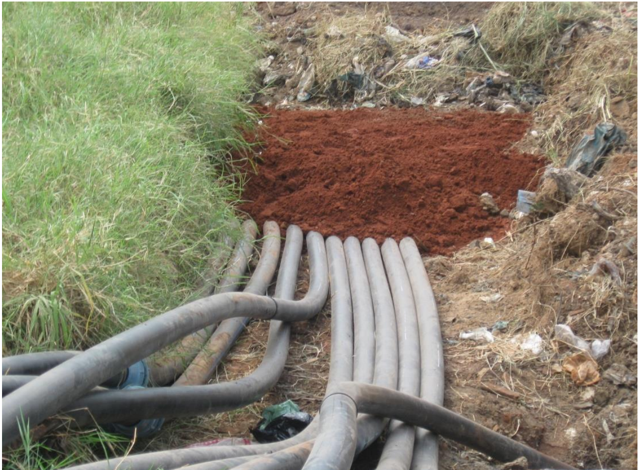
Figure 15: Multiple Horizontal Pipe Insertions
