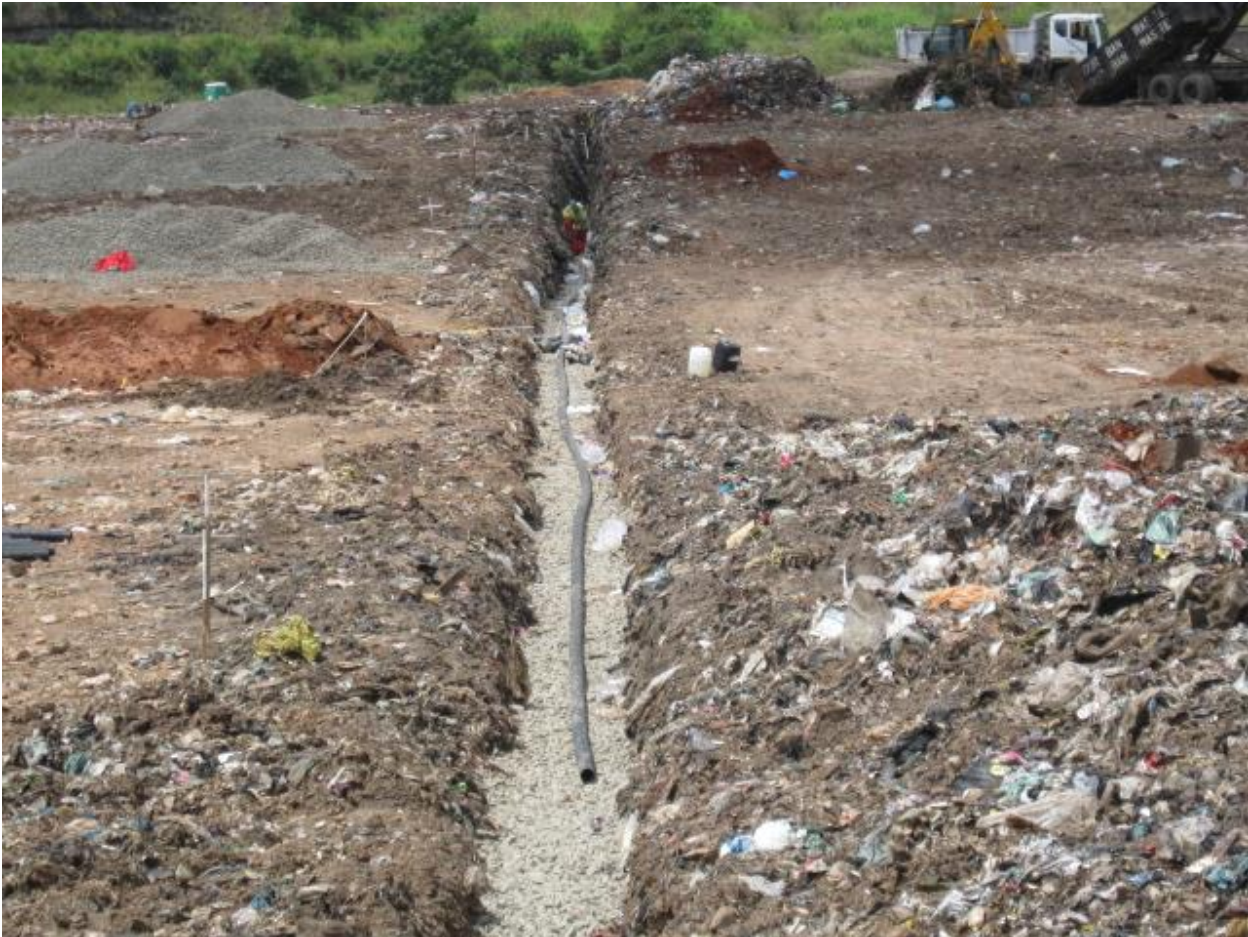
Figure 14: Typical Soil Dug-Out at Landfill Site for Horizontal Pipe Insertion
