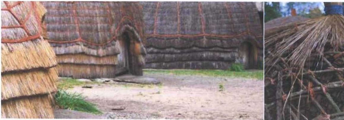
Figure 6.15: Beehive Hut structures in a village formation (left) and a typical timber structure clad with thatch (right)
