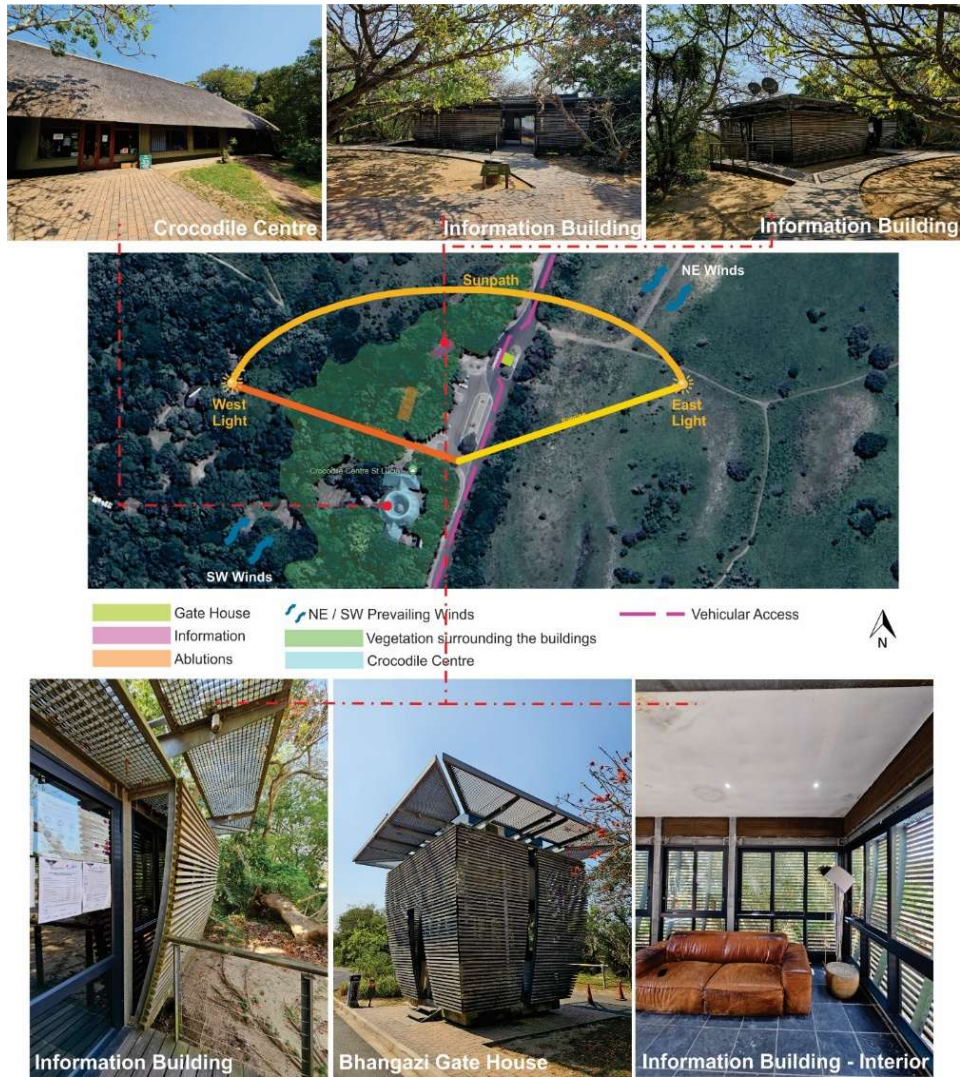
Figure 6.27: Image depicting the study site and architectural features of the Information facility and Bhangazi Gatehouse
