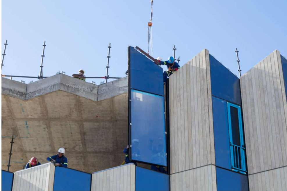
Figure 5.27: Zigzag-Shaped engineered timber facade
