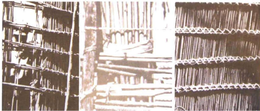
Figure 6.8: Reed panel construction
