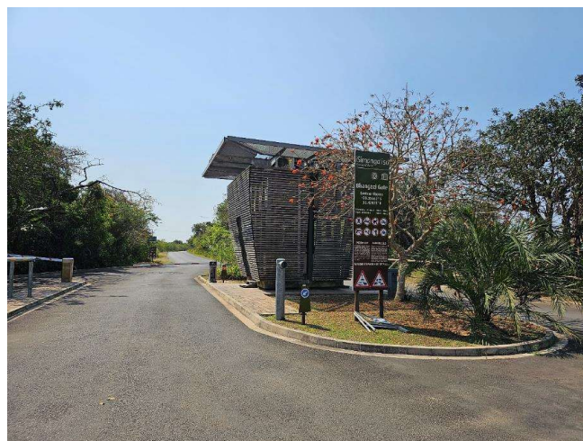
Figure 6.24: Image of the Bhangazi Gatehouse at the entrance of iSimangaliso Wetland Park, and access into the Eastern Shores
