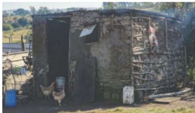
Figure 6.20: Photograph of a house made of sticks, reeds and mud in the Mtubatuba Village
