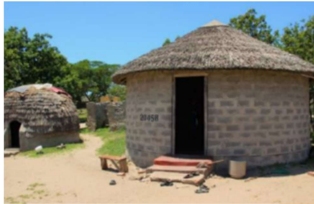
Figure 6.21: A photograph of a hut made from concrete blocks, with an adjacent hut made from seamless thatch
