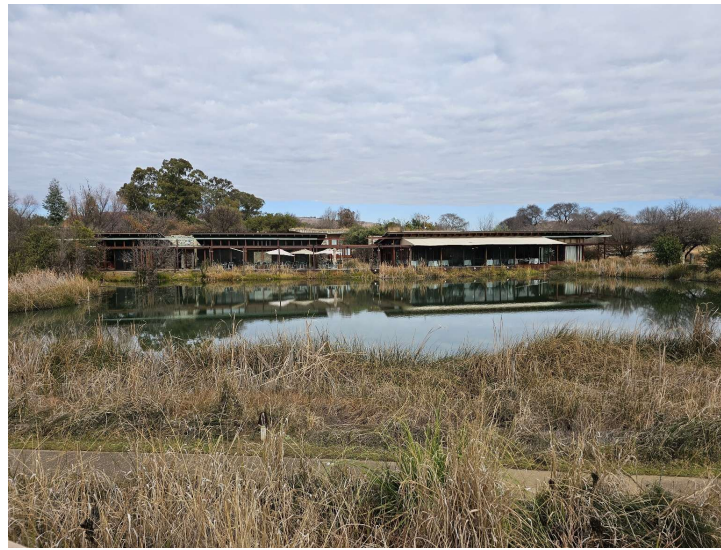
Figure 5.10: Buildings overlooking the water body
