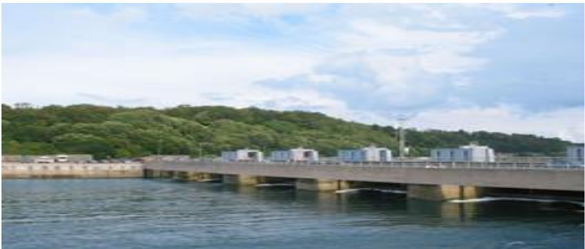
Figure 5-11: Barrage of the tidal power plant on the estuary of the Rance River in Bretagne, France
