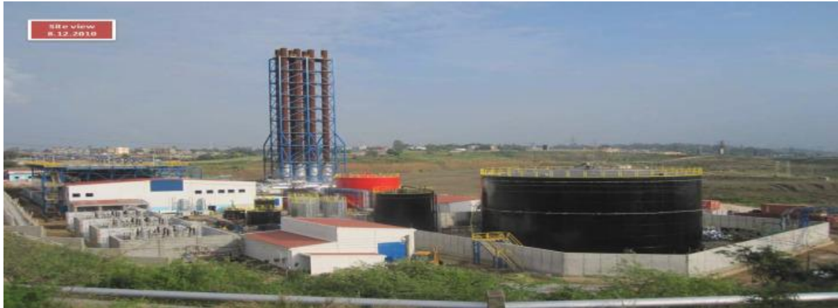
Figure 5-1: An operating 120 MW diesel engine power plant at Kipevu Mombasa, Kenya [280]
