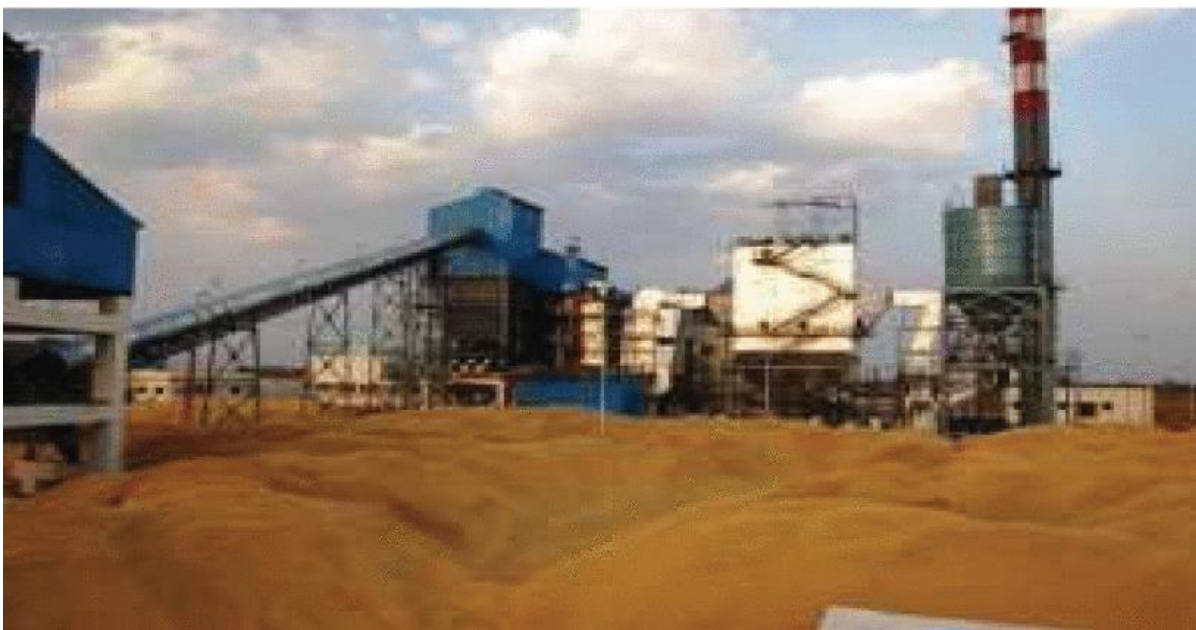
Figure 5-15: Bagasse fuel in a sugarcane bagasse cogeneration power plant
