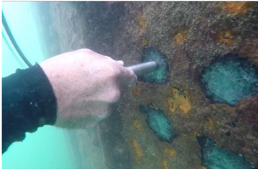
Figure 2.19: Underwater thickness measurement with an ultrasonic sensor Source: Solorzano (2018)
