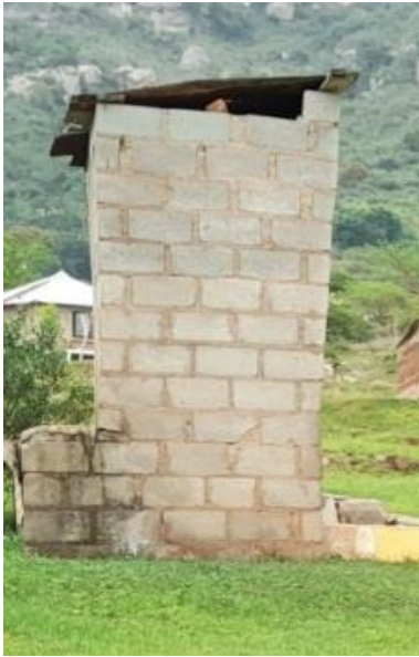
Plate 2: Self built pit toilet in Mzinyathi (Photo: S Gwala)
