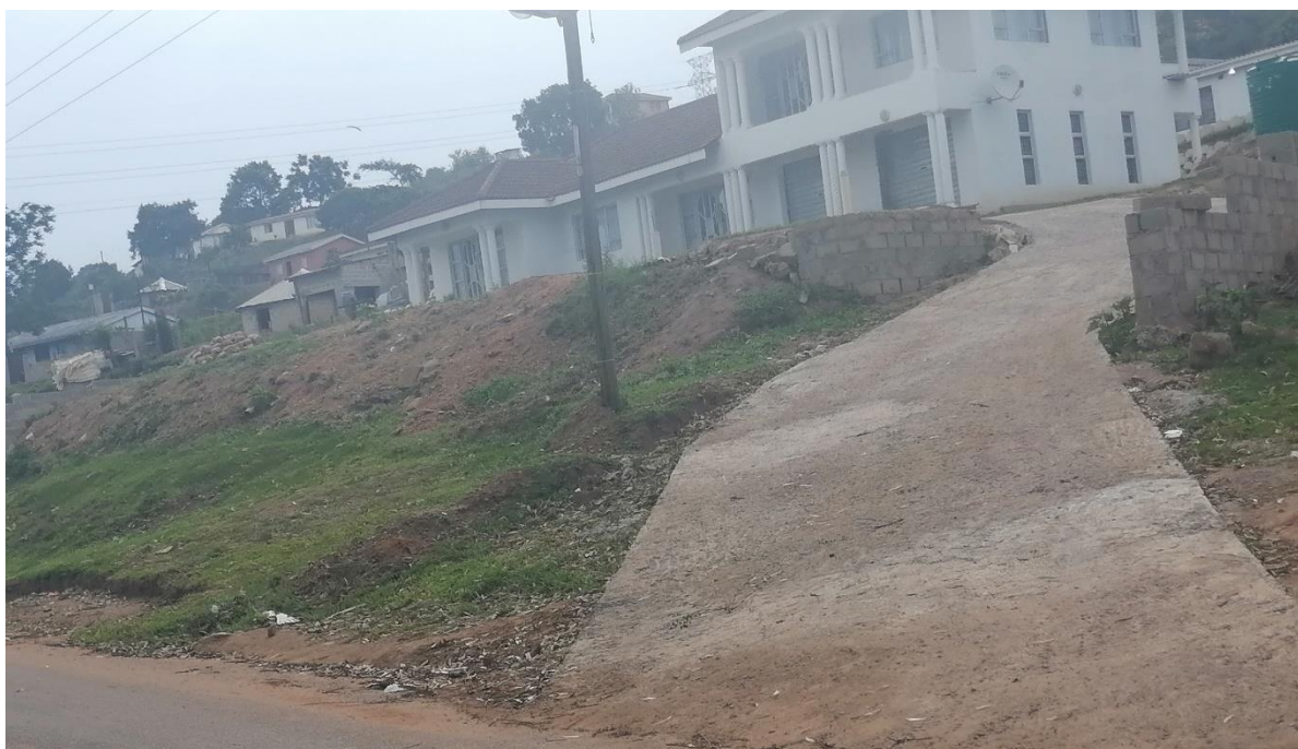
Plate 10: An example of formal dwelling houses in Mzinyathi (Photo: S Gwala)
