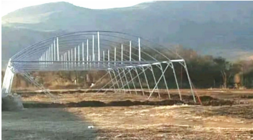
Figure 45: The structure of the Greenhouse tunnels in Mpharane village
