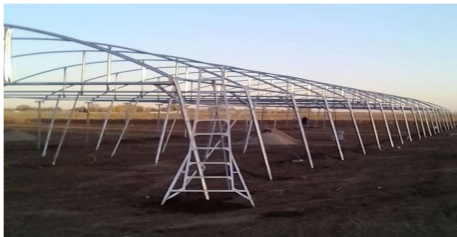
Figure 46: The structure of the Greenhouse tunnels in Maqoala village
