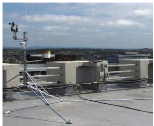
Fig. 3: an image of Existing UKZN Howard College Station.
