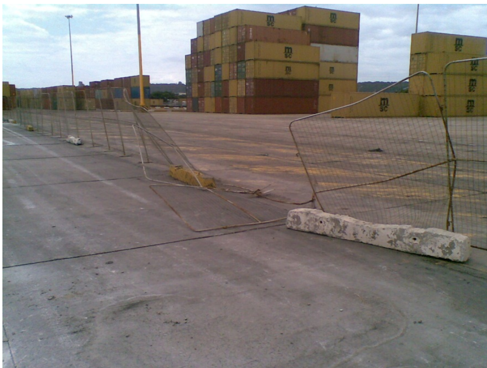
Fig 4: Fence damaged by a SC
